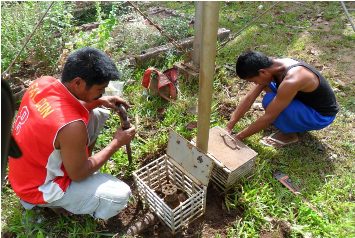
Fixing the leaked pipe.
